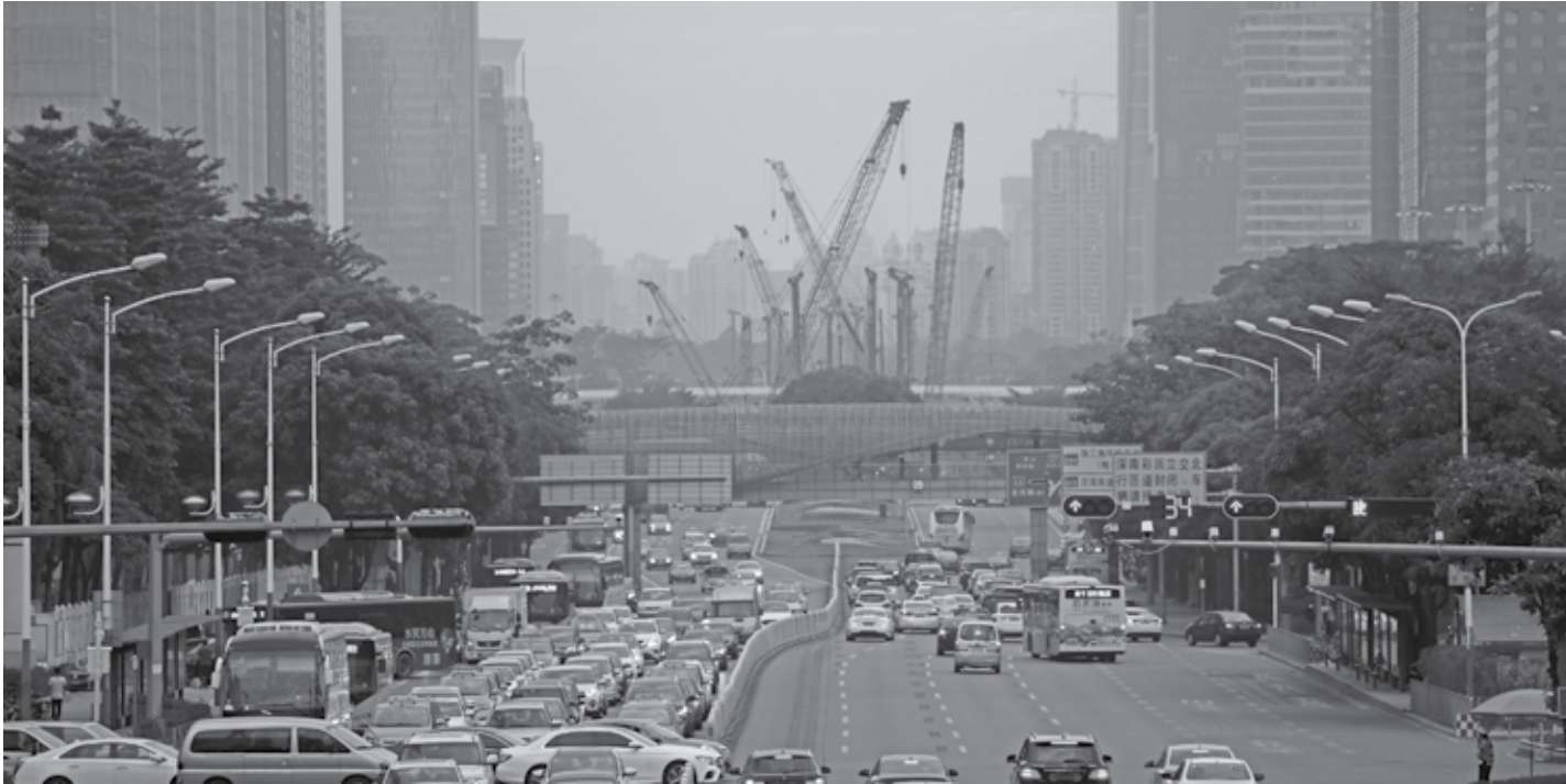
A construction site in Shenzhen in southern China's Guangdong province
